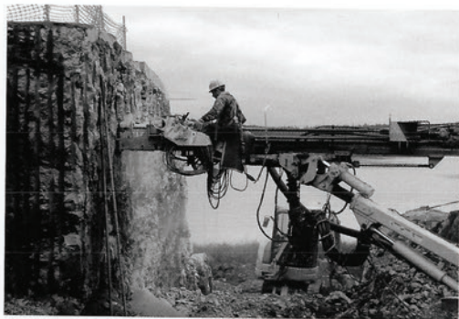
Excavating the rock at the Pierre, Lopez Island, Washington, 2010.
