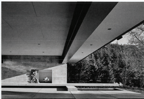
Underside of the bridge, which uses eighty-foot-long flange beams, at Whistler Ski Cabin, Whistler, British Columbia, 2015.
